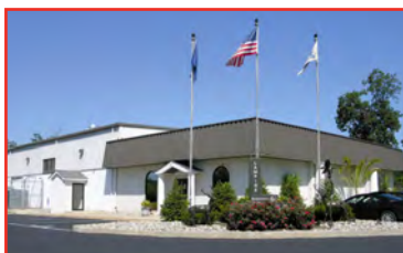
Biotech Research & Resource Center Pipersville, PA
